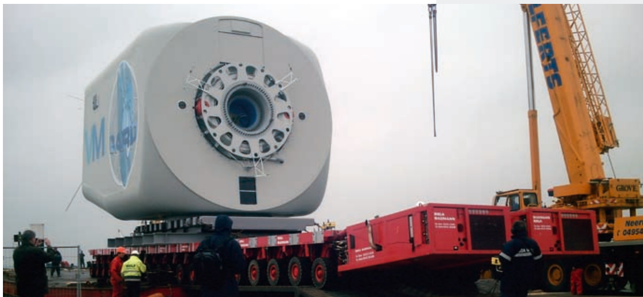
Transporting a 280-tonne BARD VM turbine generator
